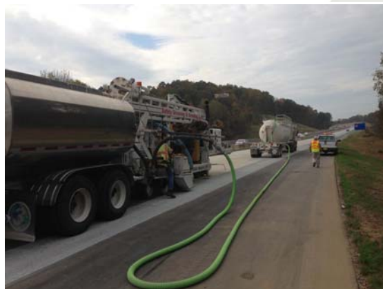
Diamond Grinding New Concrete
