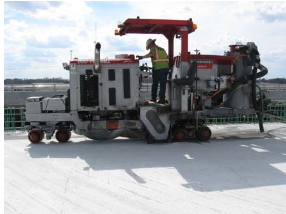
Diamond Grinding on New Bridge Deck
